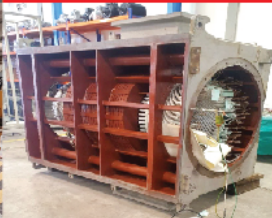
13.8 KV - 3100 KW Re-winding
